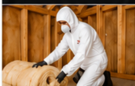
FIBERGLASS INSULATION HANDLING
